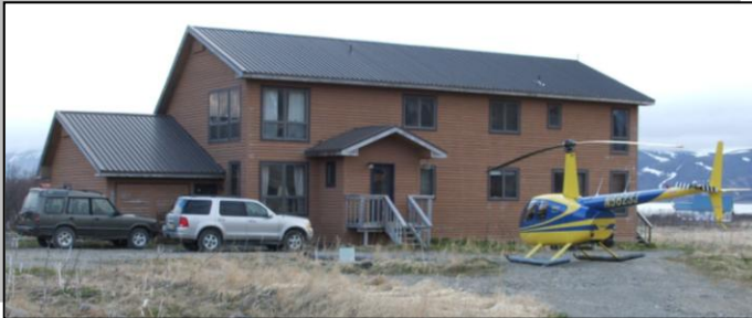
The Isanotski Corporation website will feature photos of the triplex renovation project once it's completed. Photo by Cindy Beamer.
