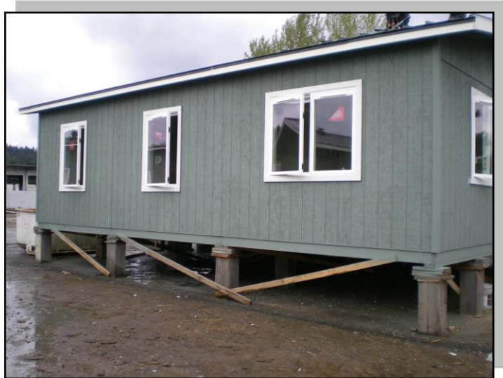
Akutan has completed the construction of three new housing units on Akun Island to serve travelers and staff at the Akutan Airport. Photo by Timberland Homes.
